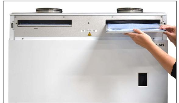
4. Remove the two filters from the ventilation unit. It is advisable to vacuum/clean the filter chambers for potential dirt, spiderwebs and leaves.
